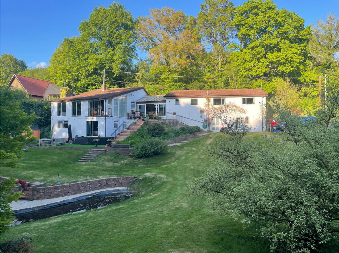
Existing House Rear Elevation
